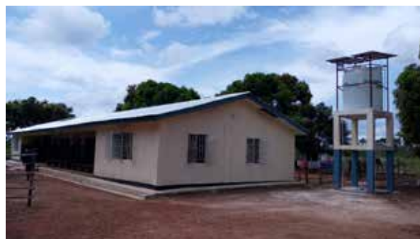
Gbanti facility after rehabilitation
