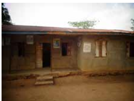
Magbafth before rehabilitation
