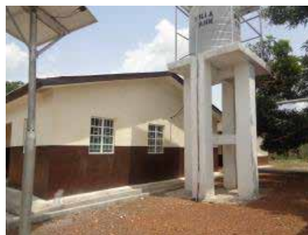
Ronietta CHP after rehabilitation
