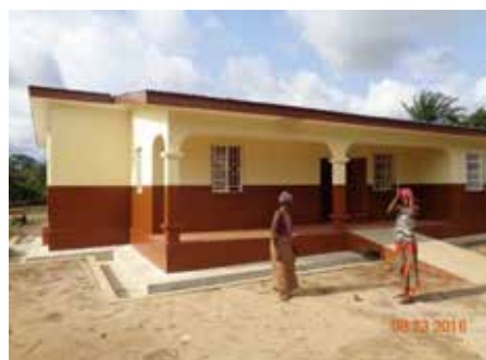
Magbafth after rehabilitation
