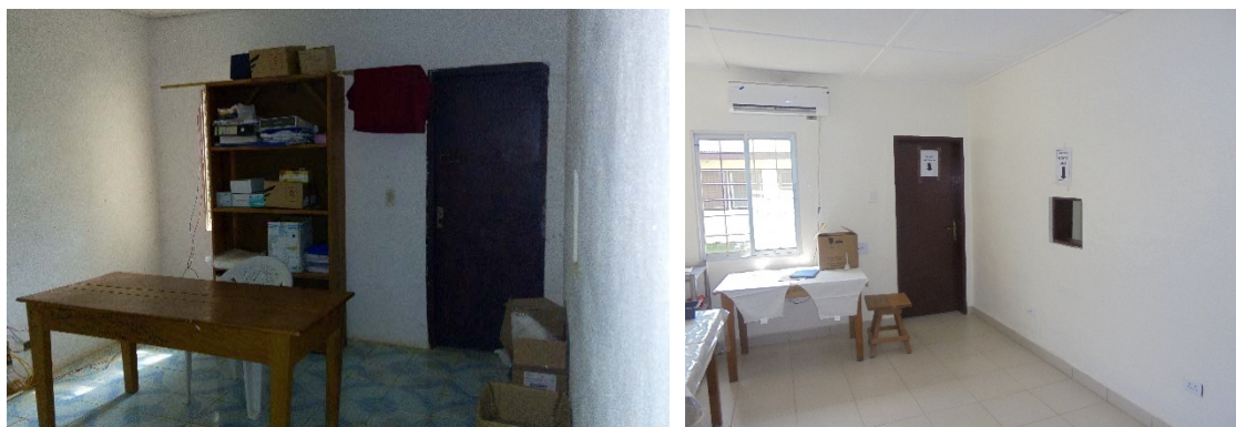
Tellewoyan specimen collection area, pre- and post-renovation. Photos: APC
