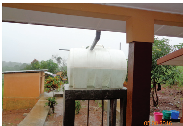
Rain-water catchment system at Tokeh Maternal and Child Health Post.
