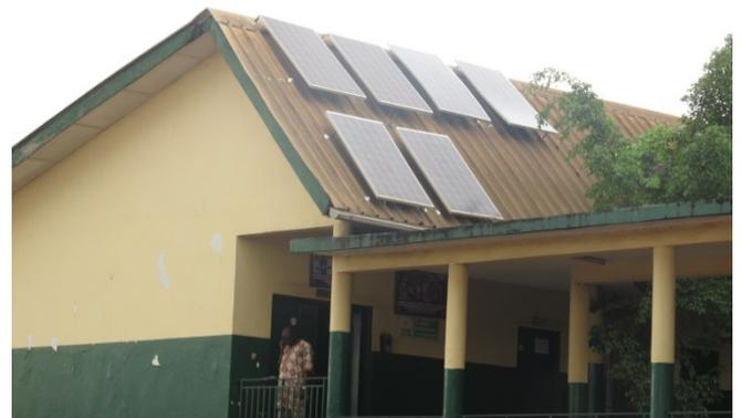
*Newly installed solar panels at Flamboyants Community Health Center ensure a steady source of electricity for the facility. The solar panels also provide power for the ophthalmology ward's slit lamp, also provided by the project. Photo: Kate Litvin, APC*
