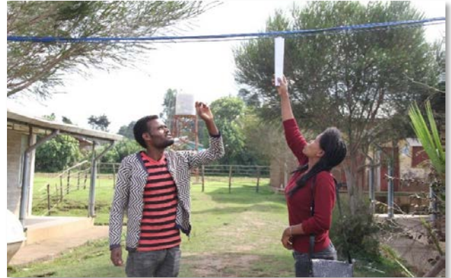
Tefera and Meskerem inspect the LAN installation at Masbira Health Center.
