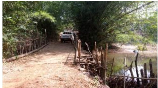
Bridge built by the community for access between Rofoindu MCHP and the city.
