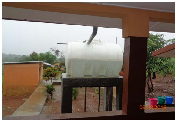
A rainwater harvesting system has been installed at the Tokeh MCHP.
