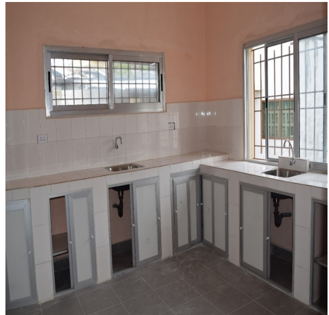
The laboratory at JFK Medical Center Outpatient Infectious Disease Clinic after renovation. Photo: APC.
