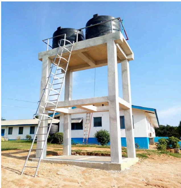
The newly constructed water tank at Kolahun Hospital. Photo: APC.
